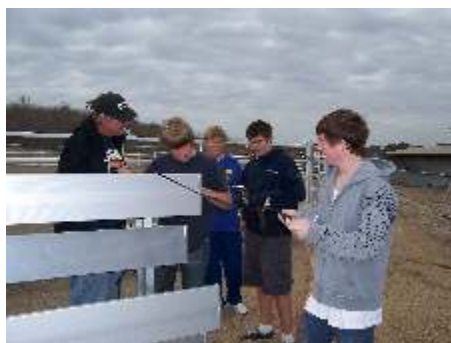
Nick (foreground) and his crew (from right to left) Zack Zombeck, Brett Kubon, Brent Spaulding put on the finishing touches.
